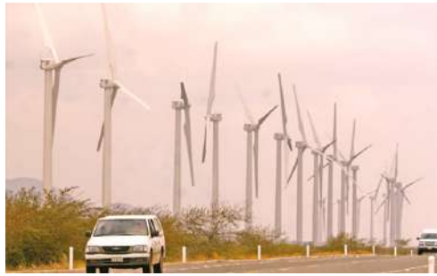
Figure 1.7: Wind farm Dominica in San Luis Potosi [10].
