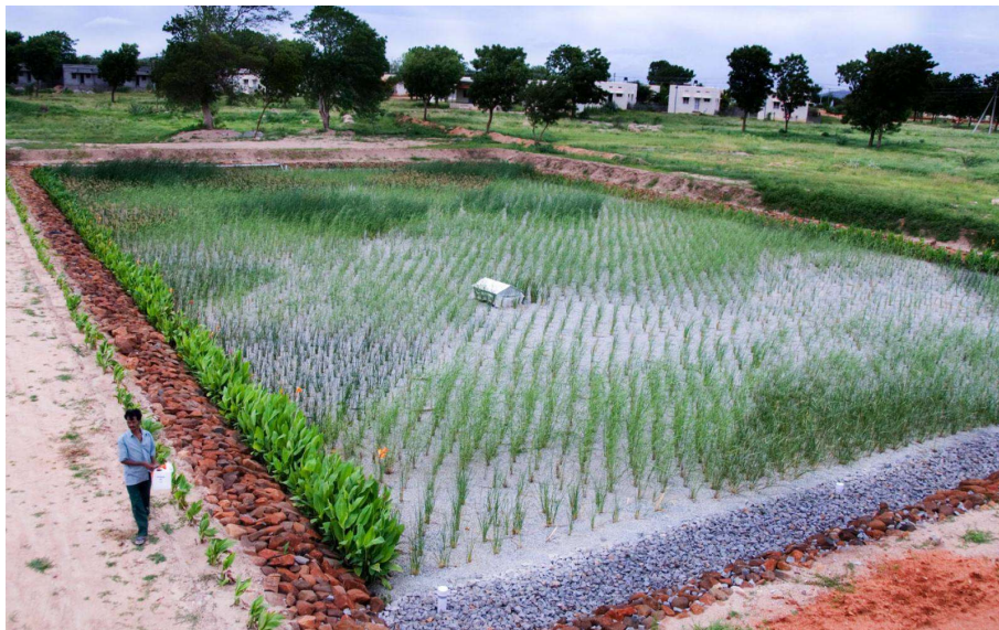
Figura 3-10 - Humedal artificial, (Iagua, 2016)
